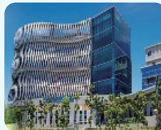
Kaohsiung Municipal Cijin Hospital
